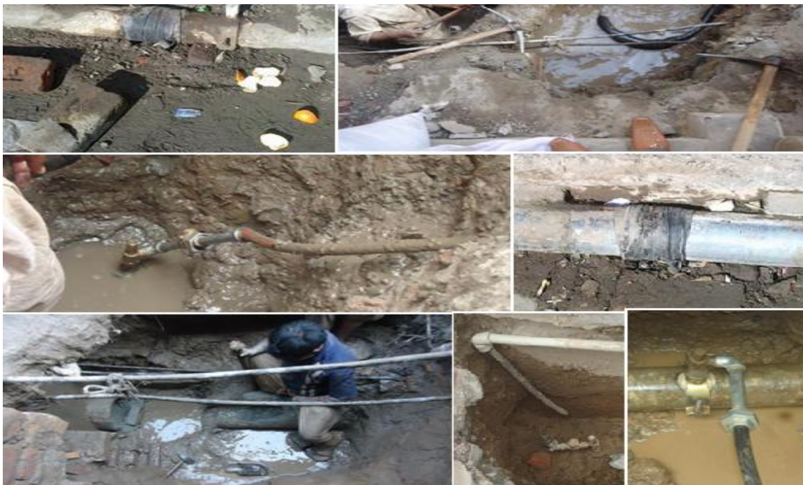
Fig 14: Leaks repair and appropriate fittings in Faisalabad during Leak Detection
