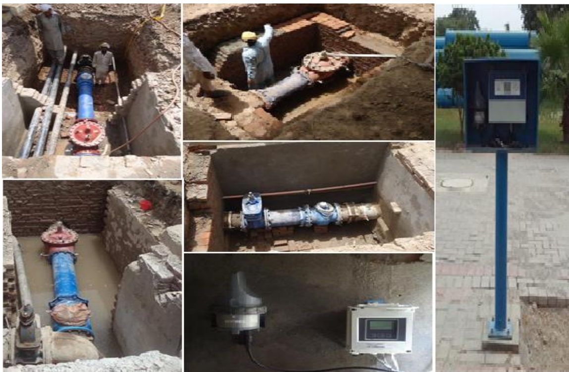
Fig. 15: Installation of 3 Ultrasonic Flow meters, 2 Endress/Hauser Level Sensor and linkage of Sofrel GPRS Data Loggers with SCADA
