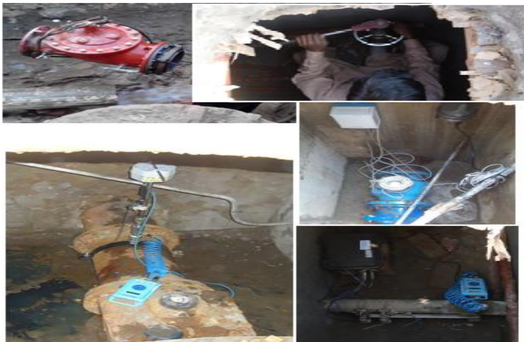
Fig. 11: Analysis of leak detection and flow measurement in Faisalabad Table 7: Results of Leak Detection and Leaks repaired details with respect to DMZ
