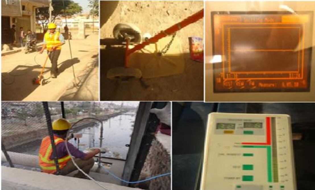
Fig. 13: Site experiment using Leak Detection Devices
